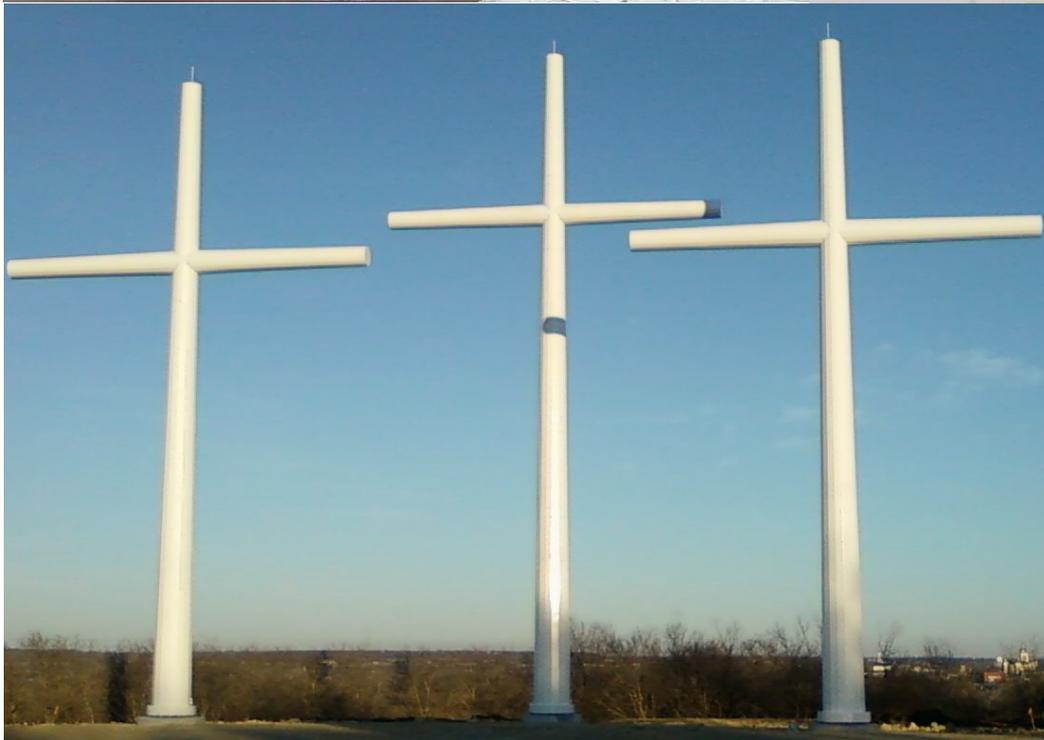
Ehresmann Engineering Cross Poles offer aesthetic characteristics pleasing to the church community. These poles have concealment sections made of plastic and fiberglass materials that are RF friendly. Custom designed to suite multiple carriers they come in various sizes and heights. Shrouded sections can conceal panel antennas behind cylinders or flat shrouds.
